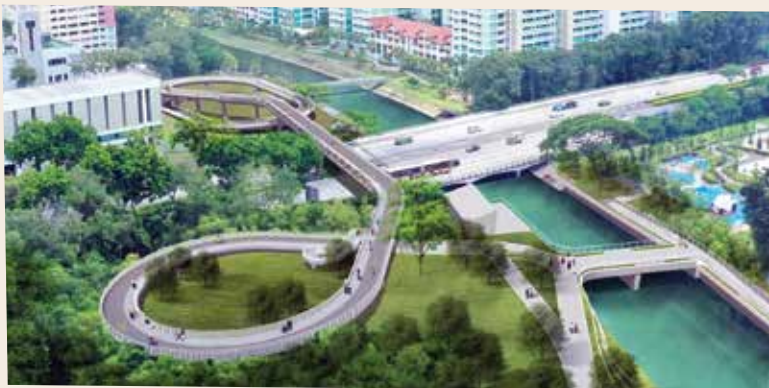
Cycling bridge connecting Tampines to Pasir Ris
