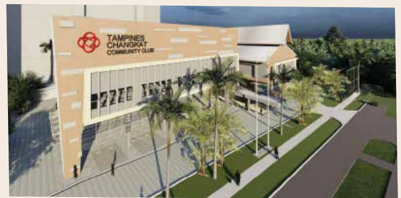
Tampines Changkat Rejuvenated Community Centre
