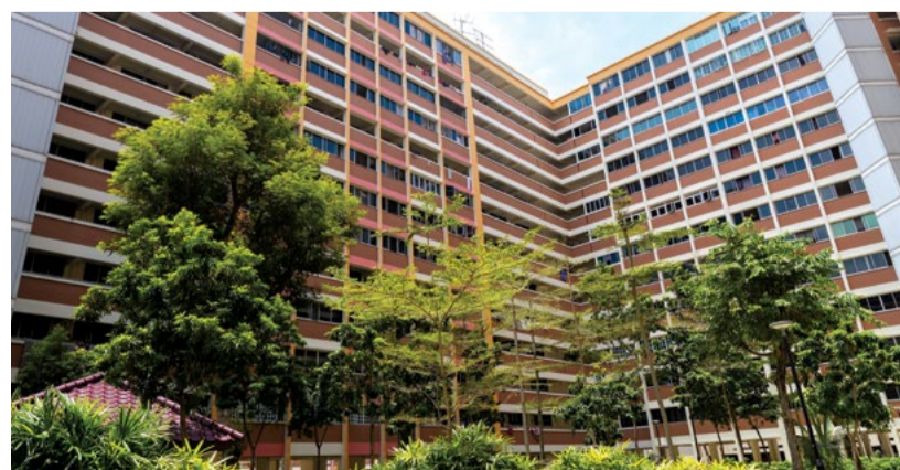
20 blocks at Tampines Street 83 and 84 will benefit from cool paint.
