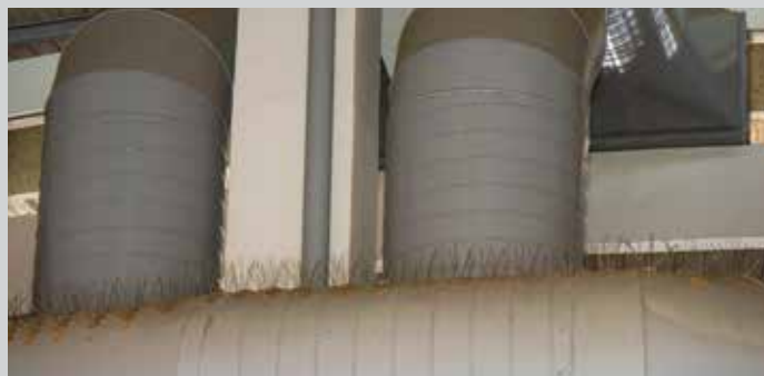
Anti-bird spikes have successfully kept most birds from entering the eating area.
