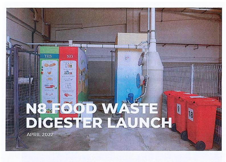
The Food Waste Digester has microbes recycling food waste into non-potable water and organic fertiliser. While the water is discharged through the drainage system, the fertilisers are distributed to merchants, community gardens, and used by Tampines Town Council for landscaping purposes.
